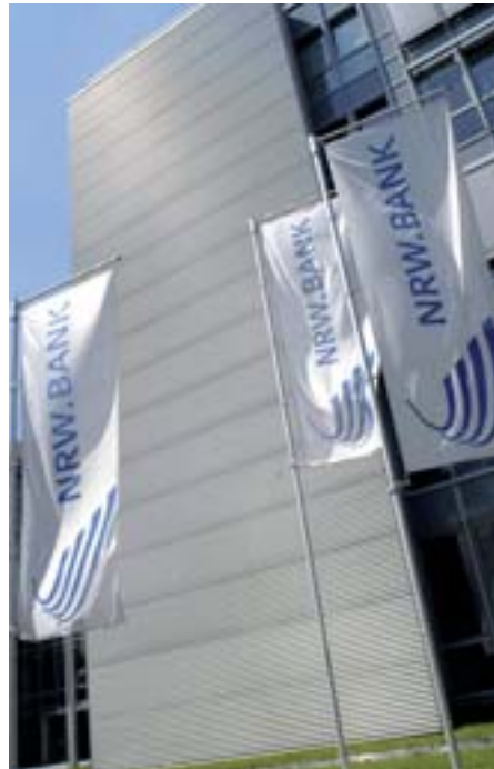
The NRW.BANK benefits from LONWORKS room automation.
