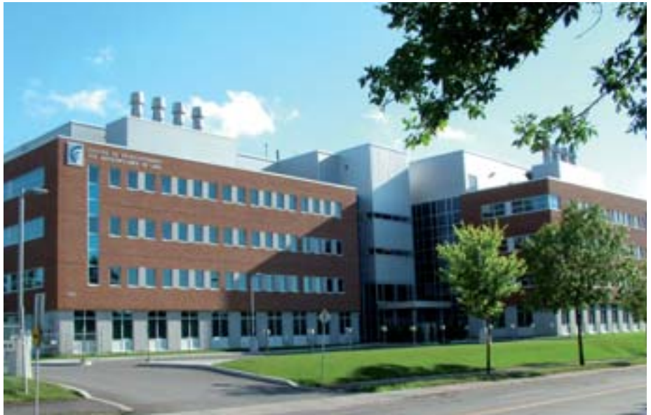
LONWORKS technology controls ambient conditions in clean rooms, labs and offices at the Quebec Biotechnology Innovation Center.
